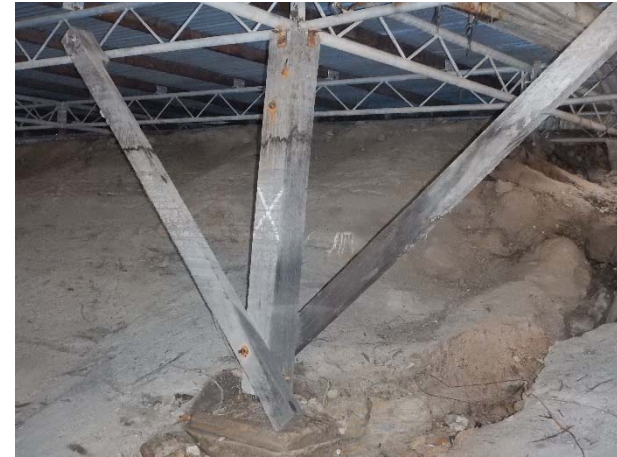
Photograph B: Typical column support and bracings on embankment
