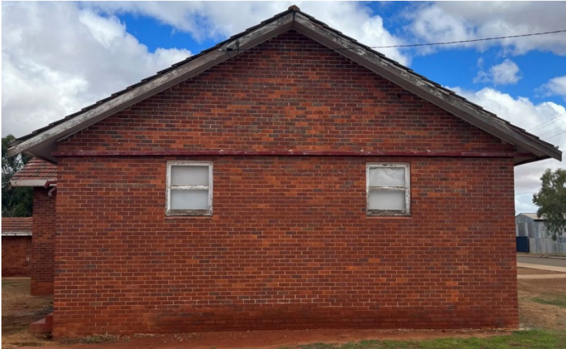
Above: West-facing wall - 43.2 m 2 (not including windows)
