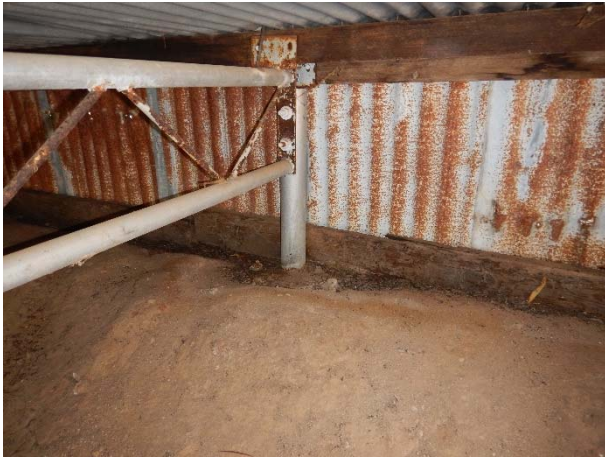
Photograph E: Perimeter support and truss
