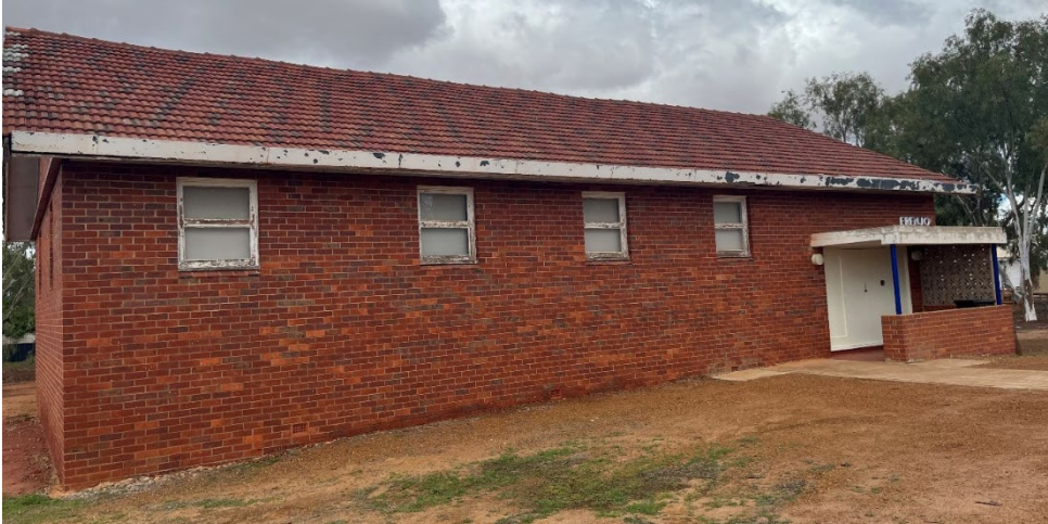
Above: North-facing wall - 40.4 m 2 (not including windows)
