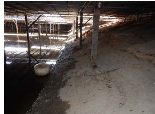
Photograph D: Accessible columns along the embankment.
