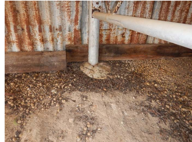
Photograph F: Steel post and concrete footing
