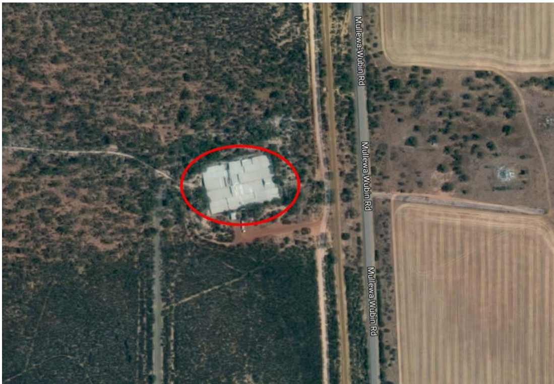
Figure 1 Caron Dam Location
