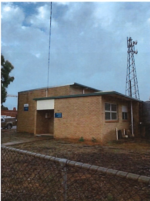
Above: Telstra building located at 32 Fowler Street
