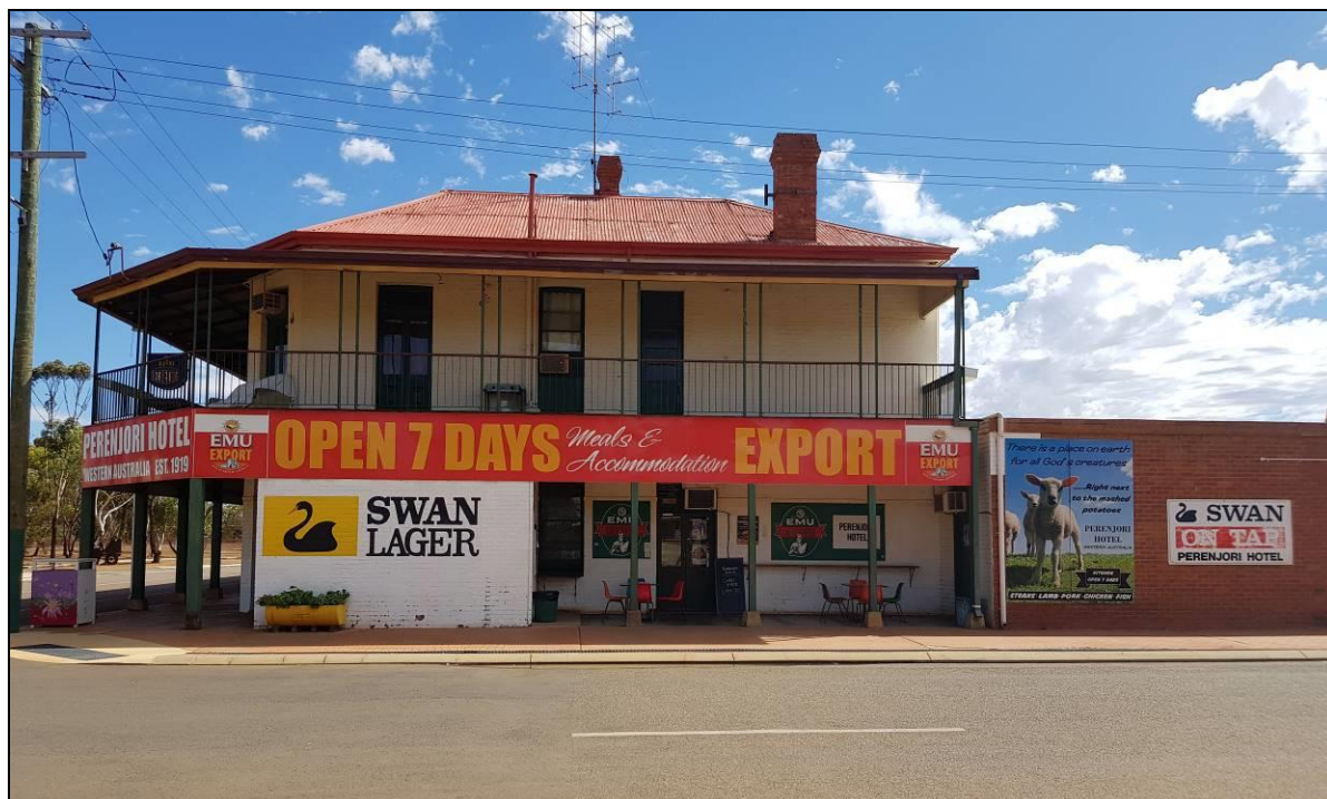
Figure 2 – View of Perenjori Hotel, Hesford Street frontage looking north-west
