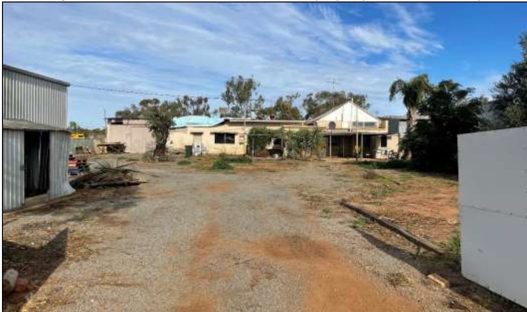
Figure 16.1(d) – View of Lot 2 Fowler Street property from rear laneway
